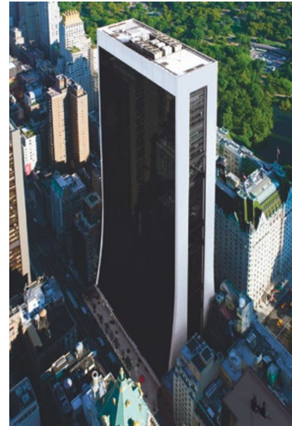
SOLOW BUILDING, 9 WEST 57TH STREET
